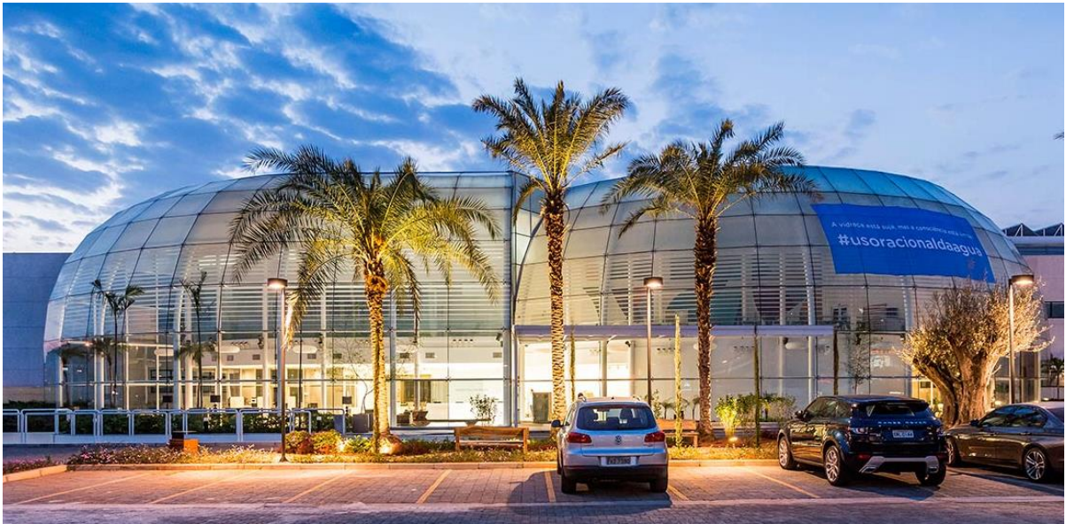
Figura 02: Fachada reformada hospital Moriah
