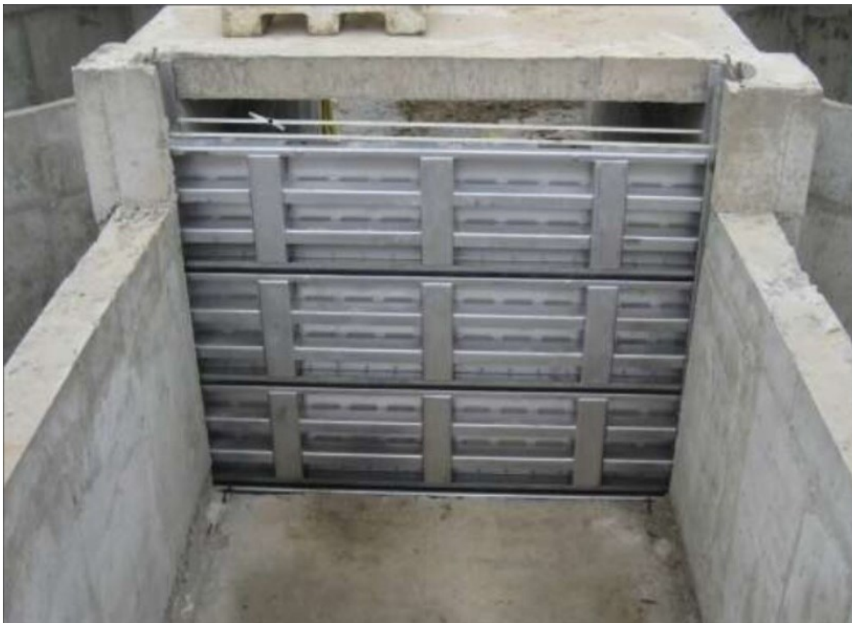
Figura 1 – Comporta ensecadeira instalada na ranhura.
