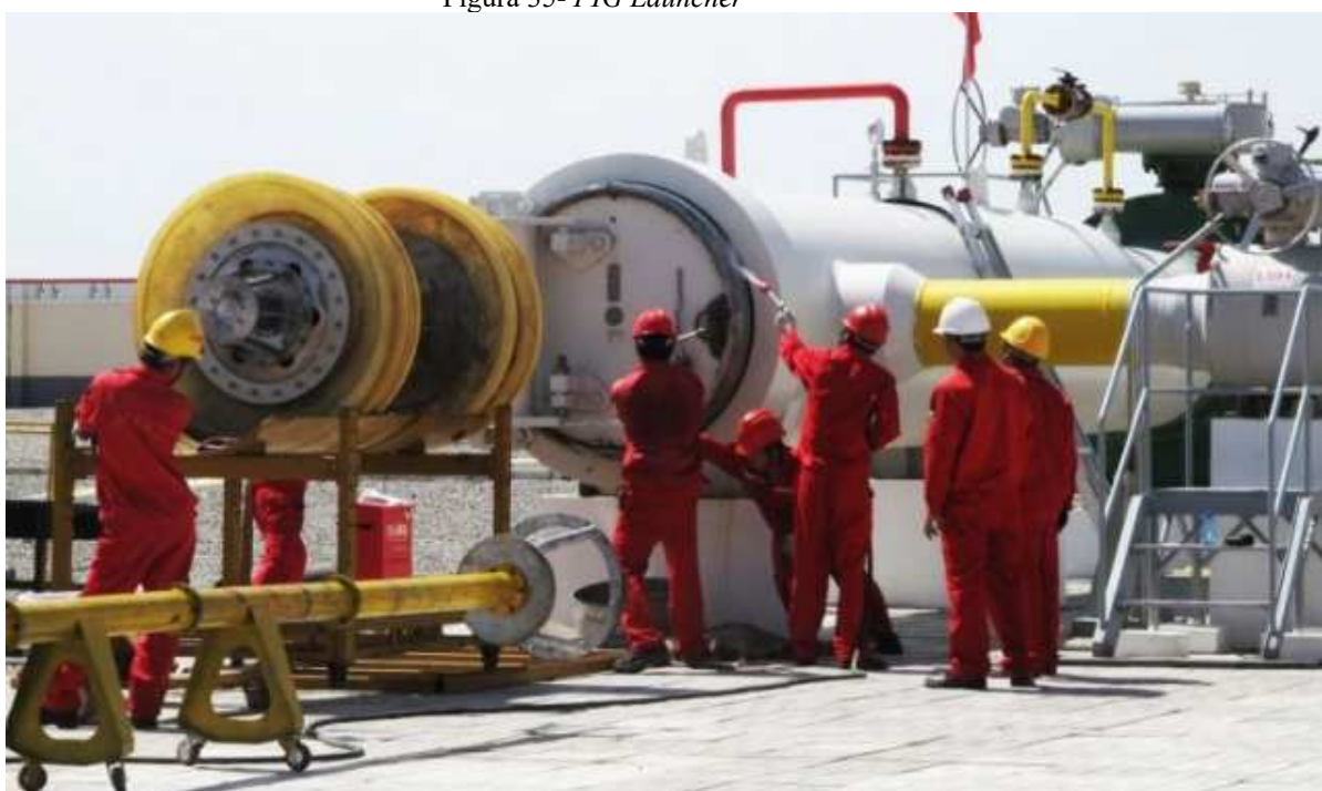
Figura 35- PIG Launcher
