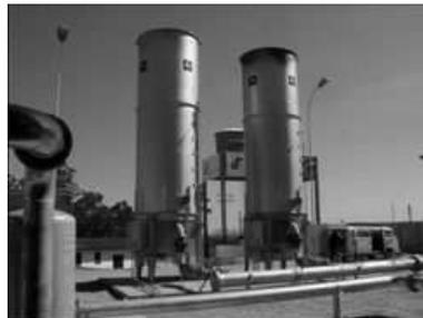
**Figure 8 - Flare used to destroy the surplus gas collected**
