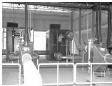
**Figure 5 - Compressors (blue) and dryers (metal)**
