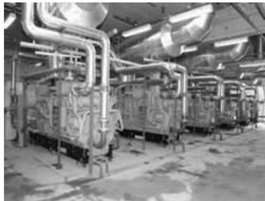
**Figure 7 - Generators used to produce electricity**
